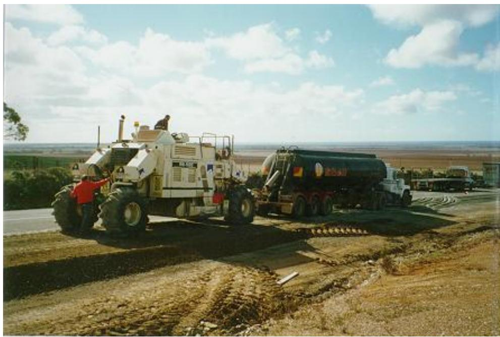
**Figure 6 Mixing Roadbond EN-1 & Water for Compaction**
