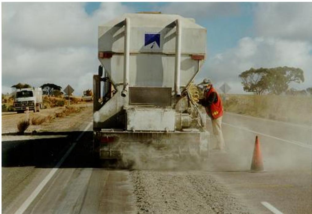
**Figure 5 Spreading Dry Binders (Flyash & Lime)**
