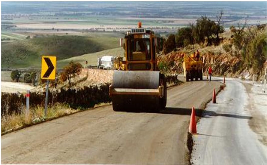
**Figure 8 Secondary Compaction with Smooth Drum & Rubber Tyred Rollers**
