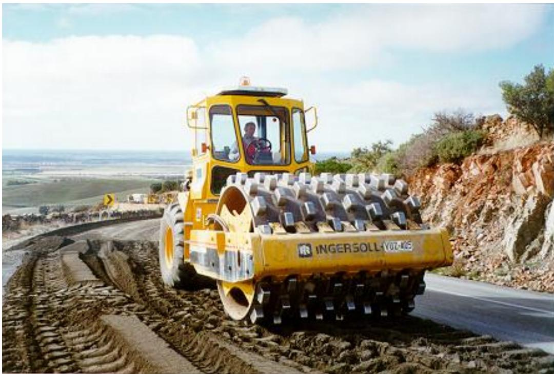
**Figure 7 Heavy Compaction with 17 tonne Vibrating Padfoot Roller**
