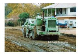
The trial sections were constructed to the same specifications with the one exception being a 50% reduction in the amount of Portland cement used and the addition of the ROADBOND EN 1. The ROADBOND EN 1 was added at the rate of one gallon diluted into 200 gallons of water per 28.5 cubic yards of pulverized roadbase mix. Once the proper amount of ROADBOND EN 1 solution was added to the material, untreated water was used to achieve and maintain Optimum Moisture Content.
